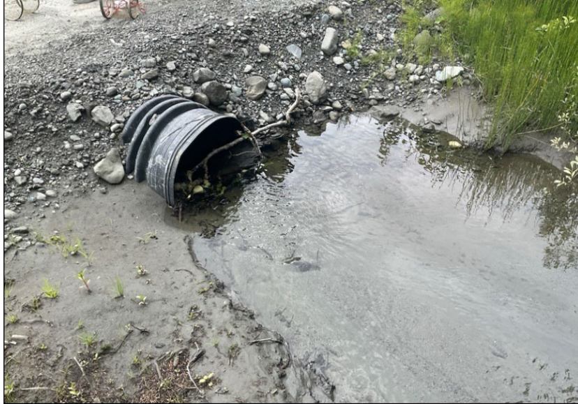
Figure 2.—Culvert inlet at waypoint 610.
