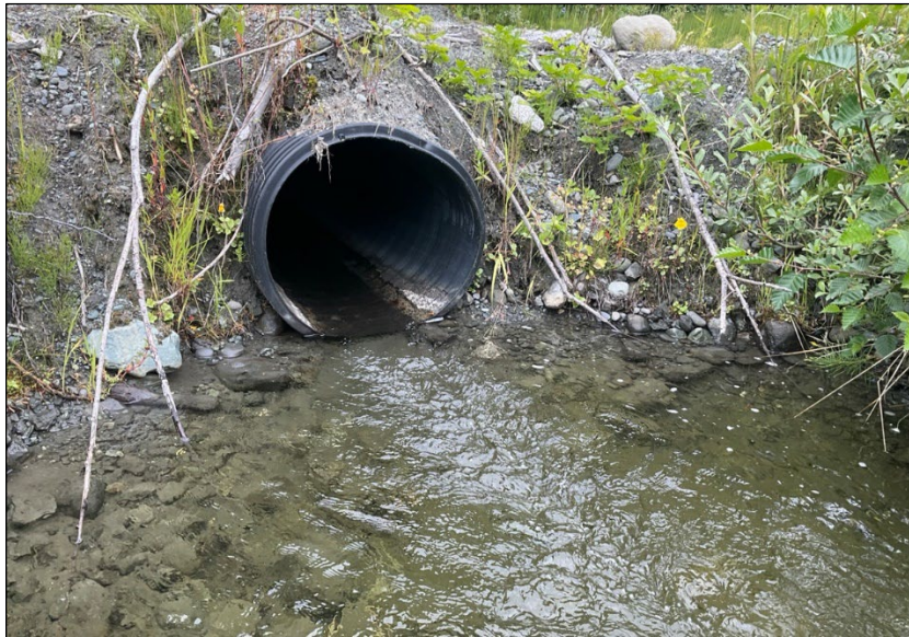
Figure 3.—Culvert outlet at waypoint 610.
